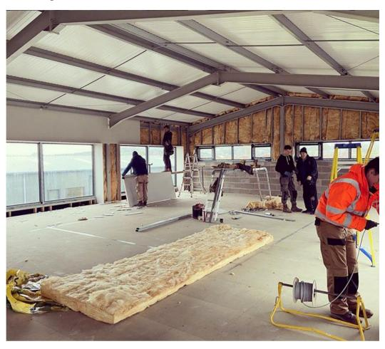
The second image shows the internal false ceiling being installed. There appears to be no sound insulation in the roof either:
